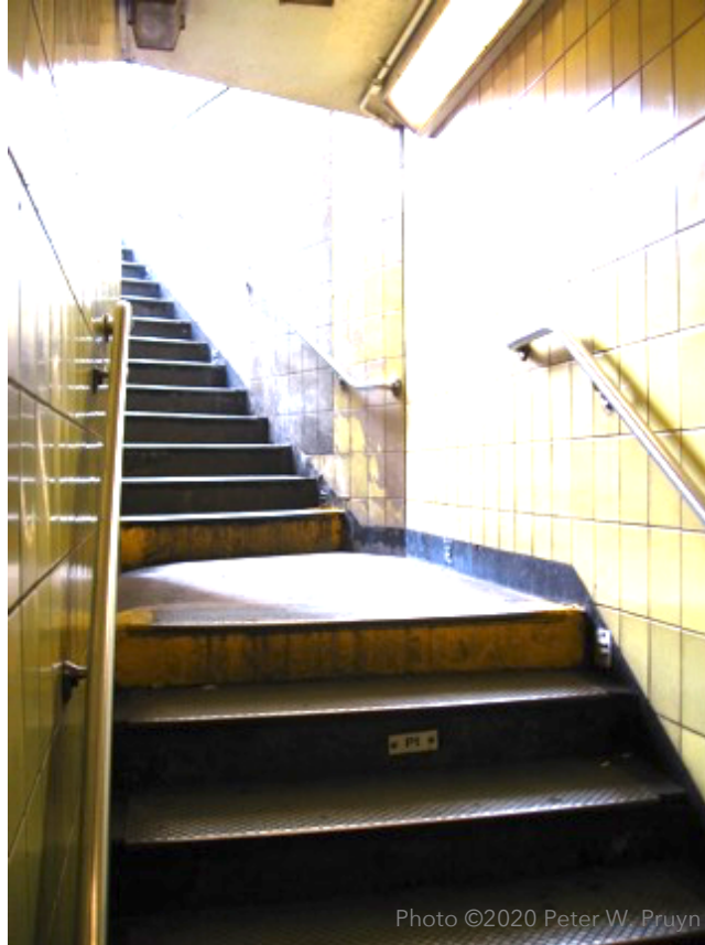
Figure 19: The subway stairs at 86th Street and Broadway.
