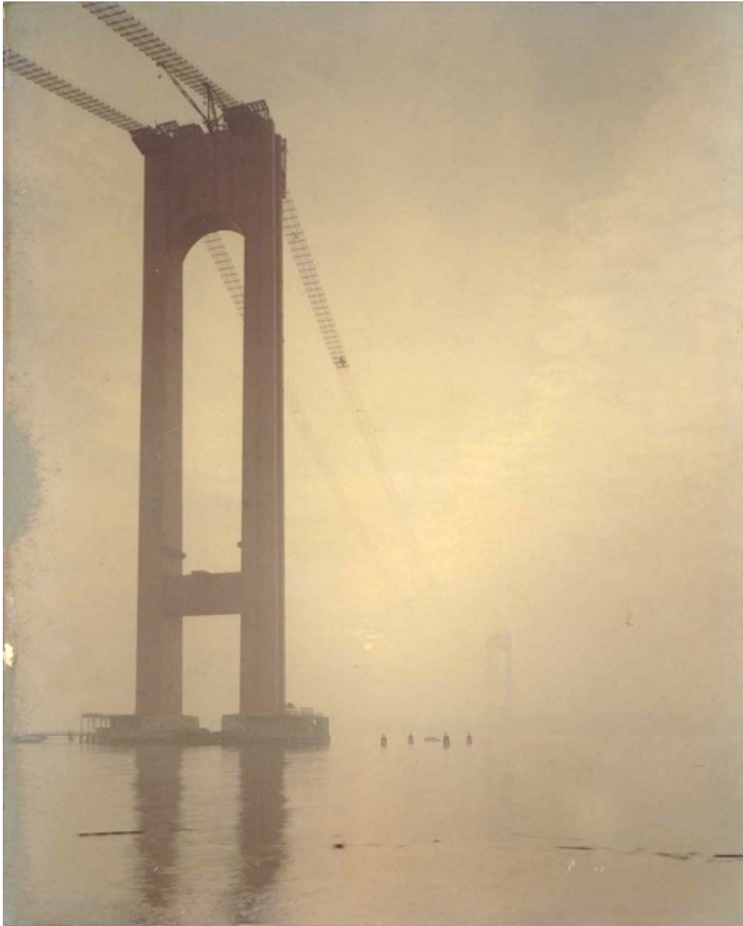
Figure 68: This photo of the Verrazzano-Narrows Bridge in New York City was taken at sunrise by my father, c.1960. The view is from the Staten Island side early in construction when only the cables had been strung between the two towers.
